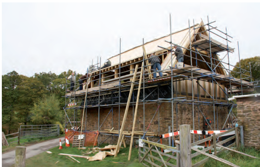
The Ruskin Studio under construction (photo: John Iles)
