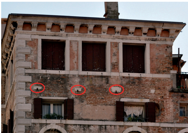
Façade showing the blocks of stone between the floors to which the tie rods are attached.
