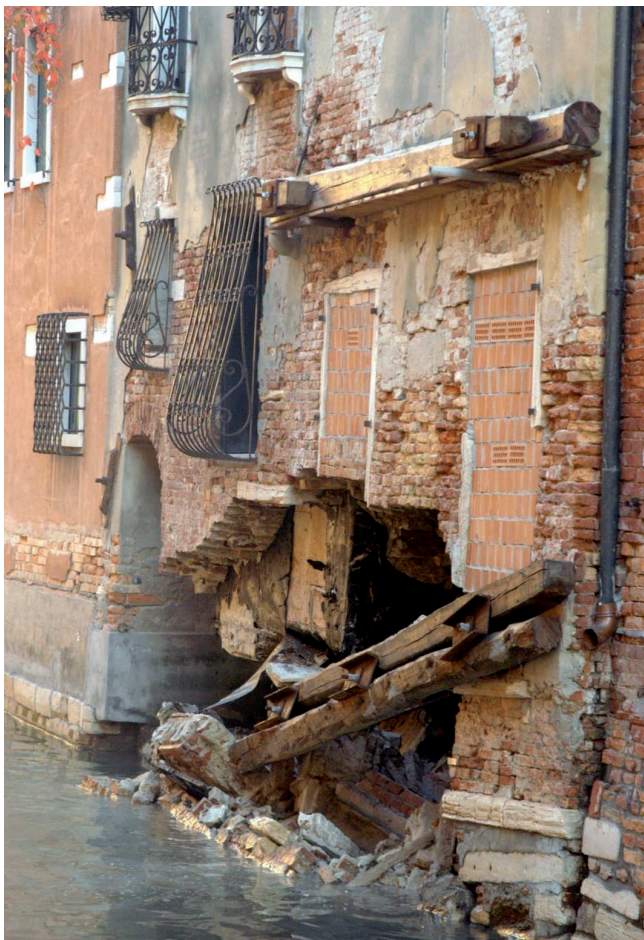
Collapse of a building near San Barnaba, 2003. The humidity in the walls caused by the rising water level will lead to the ever more frequent and dramatic episodes like this.
